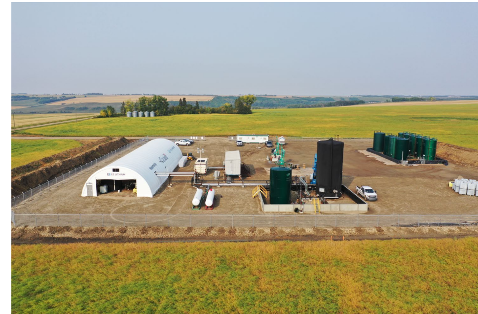
E3 Lithium’s field pilot plant in central Alberta was constructed and operated in 2023.
