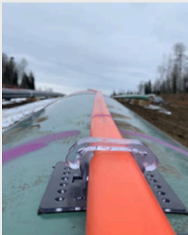
Example of FOS technology On-Pipe External Deployment
